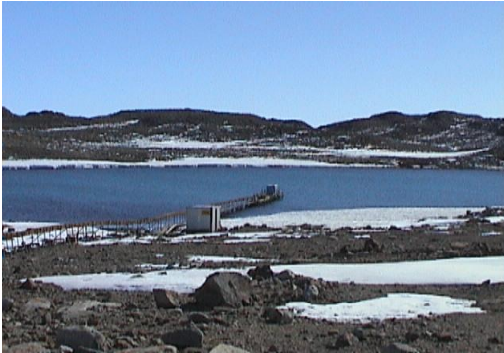
Photograph 1: Priyadarshini Lake & Pump house in front of Maitri Station
